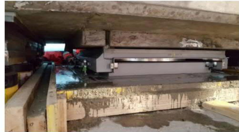
Figure 12: Grouting to the concrete substructure, welding to the steel superstructure
