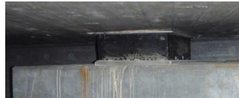
Fig.1.6.1-4: Fixed elastomeric bearing
