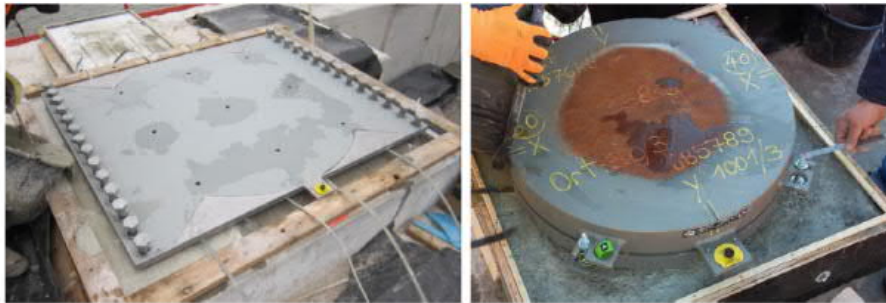
Figure 9: Underpouring of bearing, anchor plate with air outlet holes (left) and spherical fixed bearing (right)
